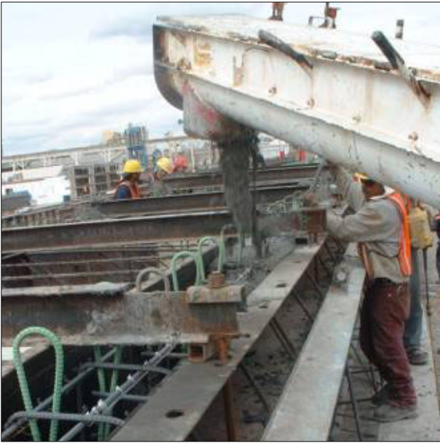
Fig. 3. SOFO sensor attached to rebar undergoing the pouring of concrete.
